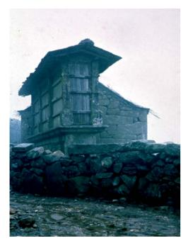
Gerês. Corn Silo. Ventilated structure used to store corn cobs. These structures of rural architecture have a very expressive presence.
